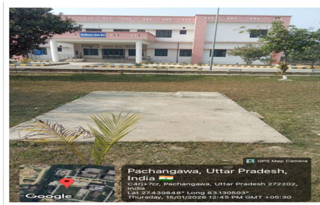
Surface Runoff Harvesting System in front of campus hospital
